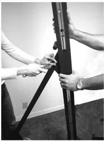
With another person holding at a slight angle, assemble the brace and tie to the post.
