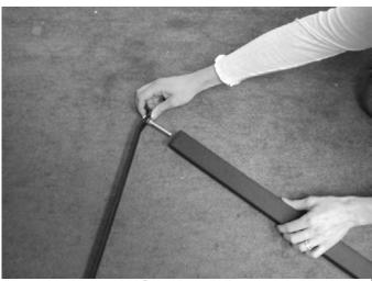
Assemble brace and floor tie together.
